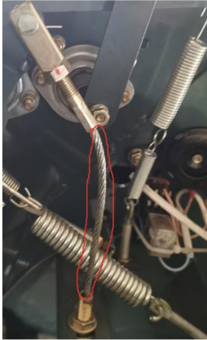
One end of the pull line
